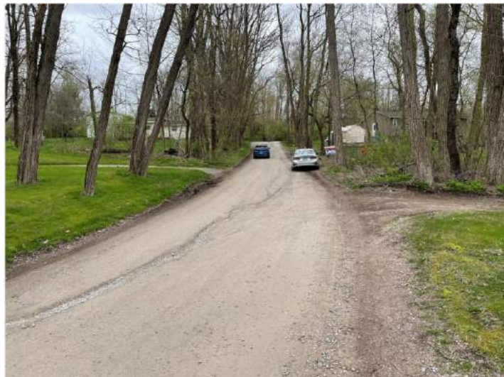
Figure 2 – Existing Roadway – Merrill Drive at Carmer Road
